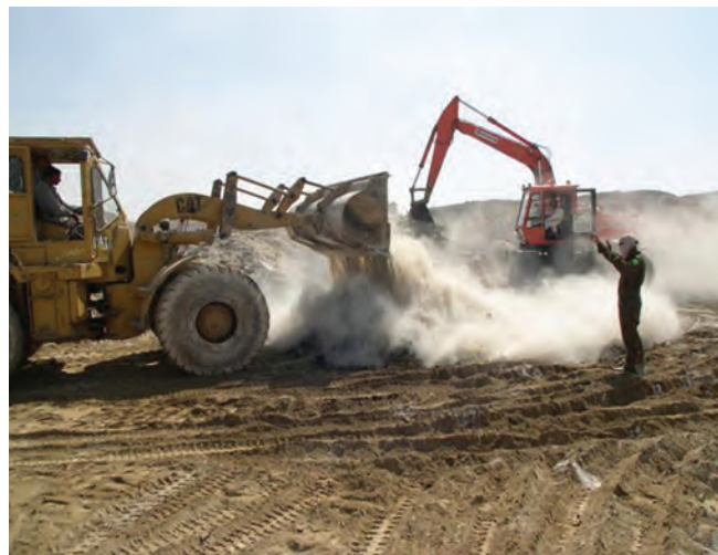
▲ Figure 18: Stabilisation of oily waste using quicklime.
