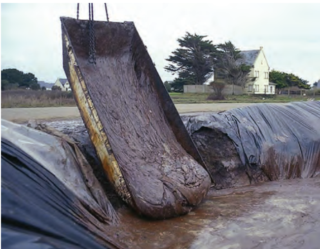
▲ Figure 11: Skip emptying emulsified fuel oil into a lined temporary storage pit.
