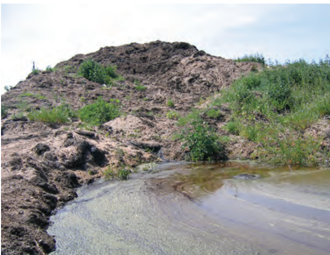
▲ Figure 13: Capture and treatment of leachate from oiled sand piled in temporary storage prevents secondary contamination of the surrounding area and groundwater.
