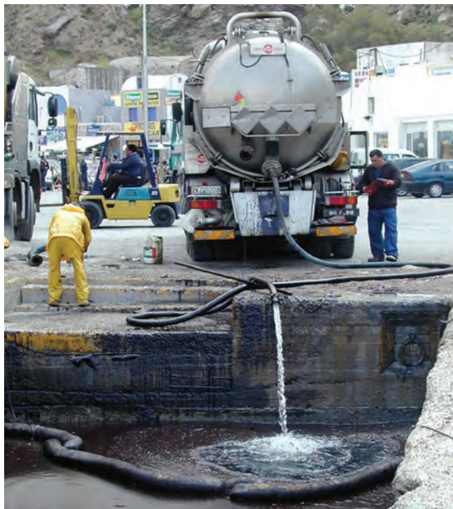
▲ Figure 15: Decanting of water into the spill area, after settling and separation of recovered oily water in a vacuum truck.
