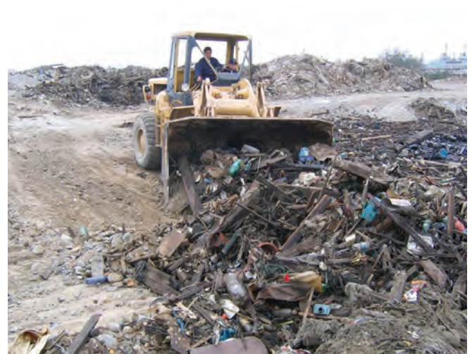
▲ Figure 14: Removing debris from the shoreline before oil strands will help reduce the quantity of oiled material requiring disposal.
