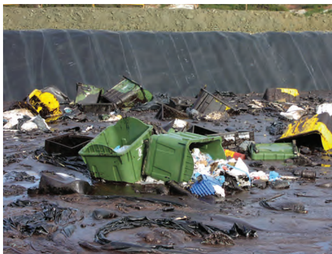
▲ Figure 9: A well-lined pit containing poorly segregated waste, requiring considerable additional effort to separate and treat.
